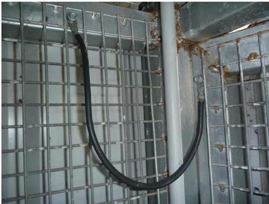
Photo 1. Example of a bond wire
