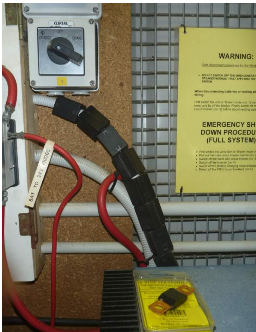
Photo 2. Setup of mains RFI filters on mains power lead
